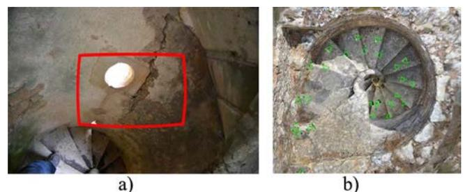
Fig. 2. a) Fisheye lens versus 18mm lens (red limits). Notice the leg size relative to the width of the step. b) Camera positions.
